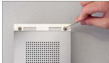
3 Connect and fix the door intercom station
